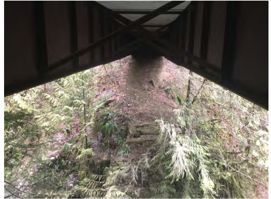
Left Bank Abutment when facing downstream
