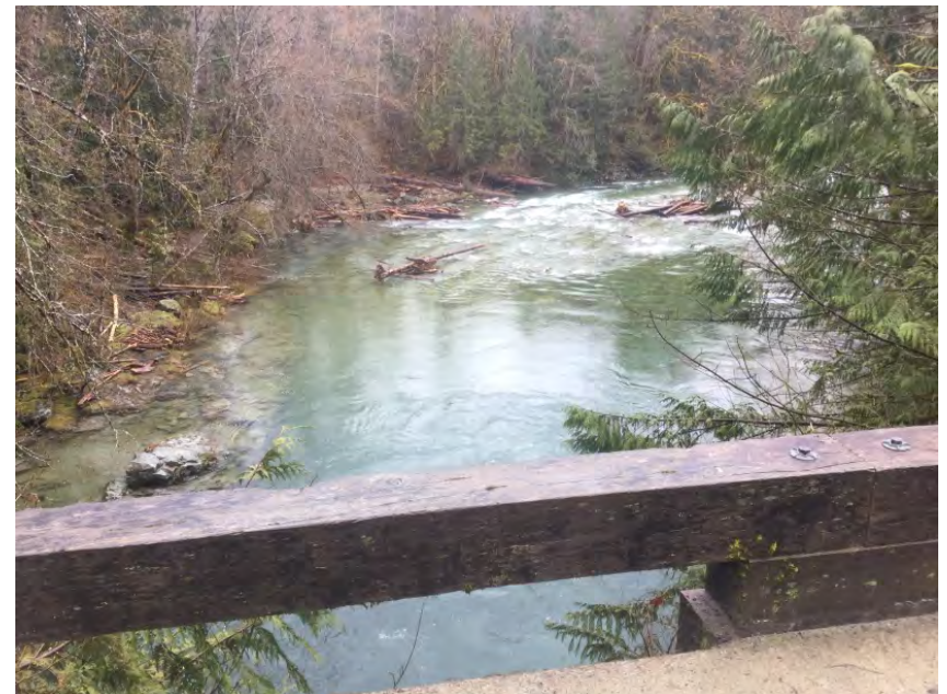
Looking downstream from deck
