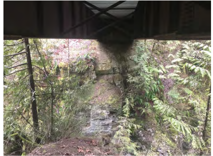
Right Bank Abutment when facing downstream
